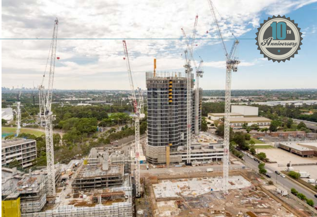
High strength tower sections allow these Terex CTL 430 luffing cranes to achieve high freestanding height on these projects.
