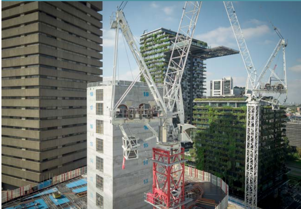
High strength tower sections allow these Terex CTL 430 luffing cranes to achieve high freestanding height on these projects.
